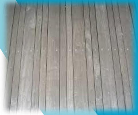
*Highly versatile, Grey Ironbark is extensively used for external applications such as cladding, battening, decking & posts as well as for internal flooring.*
