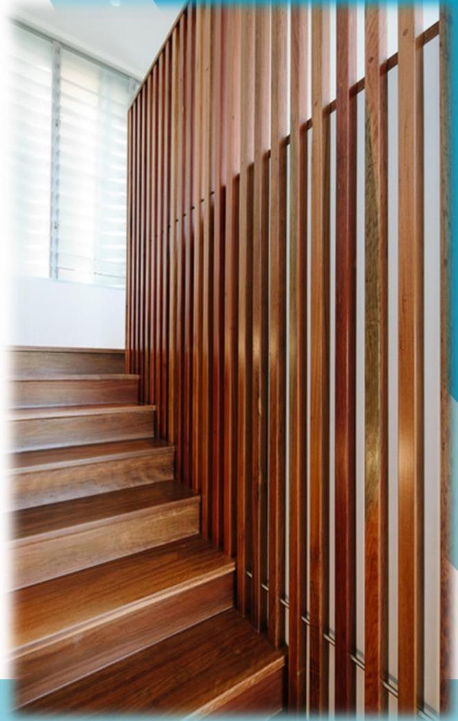
*Brush Box exhibits rich colour tones and is a visually stunning timber adding warmth and interest when combined with modern interior materials such as glass, stone and polished concrete. Its hardness makes it ideal for use as a flooring or wall panelling in areas that see a lot of traffic or where it has to take the occasional bump.*
